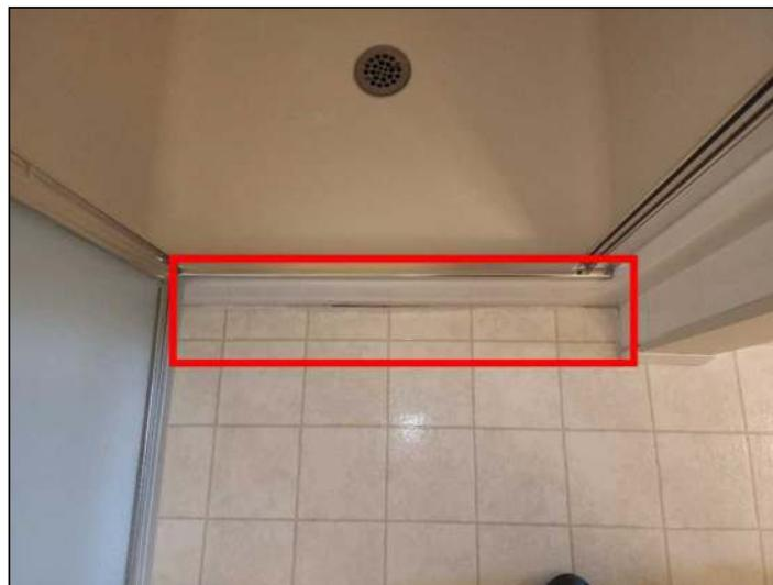
The joint along the shower and the floor needs to be sealed to prevent moisture penetration. Have a contractor evaluate and service as needed.
