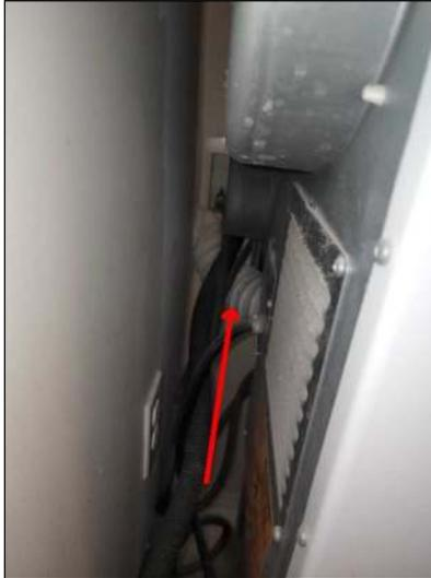
Recommend replacing flexible dry vent pipe and run continuous solid metal pipe. Install solid metal pipe with foil tape, NOT screws or duct tape.
