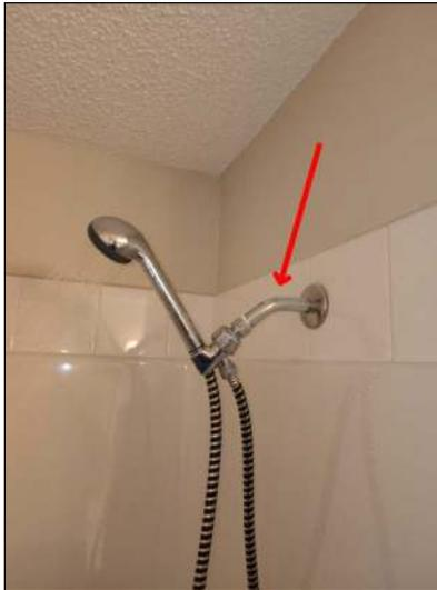
Shower mast is loose in the wall. Recommend securing properly to the wall.
