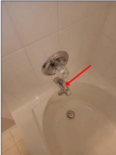
Faucet is loose in the wall. Recommend securing properly to the wall.
