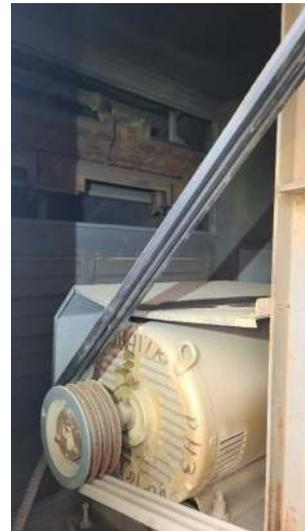
The exhaust systems are very dirty and should be serviced by a contractor accordingly.
