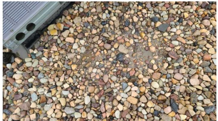
Debris blocked downspouts observed, suggest cleaning gutters and downspouts, which should be a regular part of maintenance.
