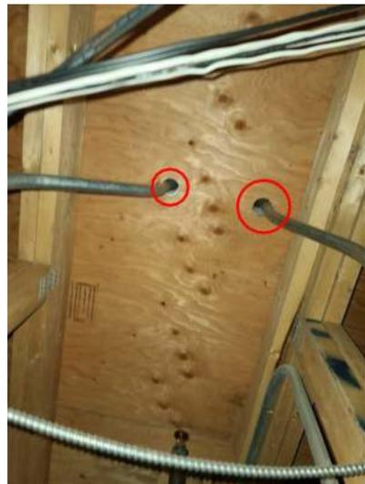
There are pipes penetrating thru the roof that need to be insulated inside to keep the hot and cold air away from each, if not serviced this can cause condensation damage to the the ceiling inside the building. Have a contractor evaluate and service as needed.
