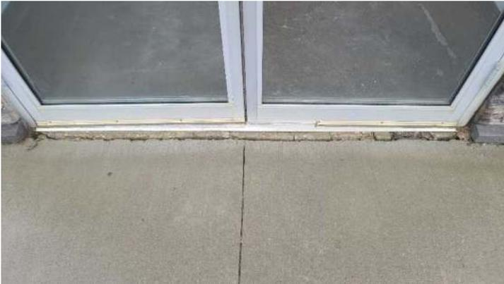
The sidewalks have typical cracks that indicate movement of the base under the sidewalk, water management needs to be addressed to control movement. If this is left it can effect the components of the building and surrounding areas.
