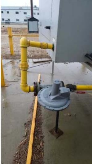
The supports for the gas piping should be evaluated by a plumbing contractor and serviced as needed.
