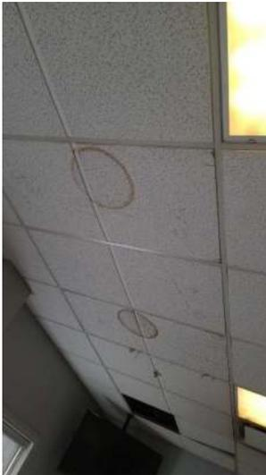
There are signs of moisture in the building that should be monitored, with the grading and drainage being poor this is a problem that may continue. A contractor should be used to evaluate the property and how to keep the moisture away from the building.
