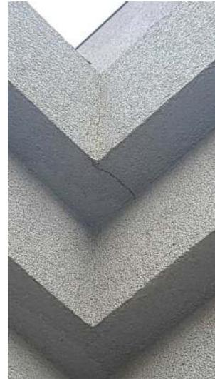
The EIFS wall covering is peeling and cracking, have a contractor evaluate and service as needed.
