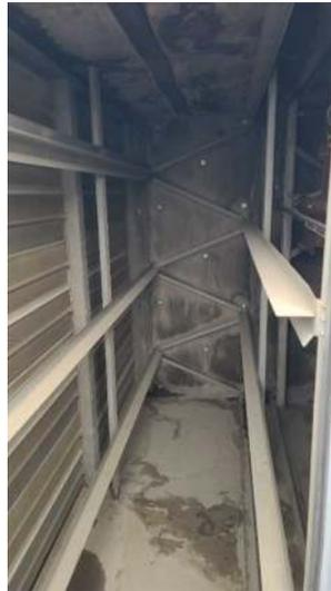
The exhaust systems are very dirty and should be serviced by a contractor accordingly.
