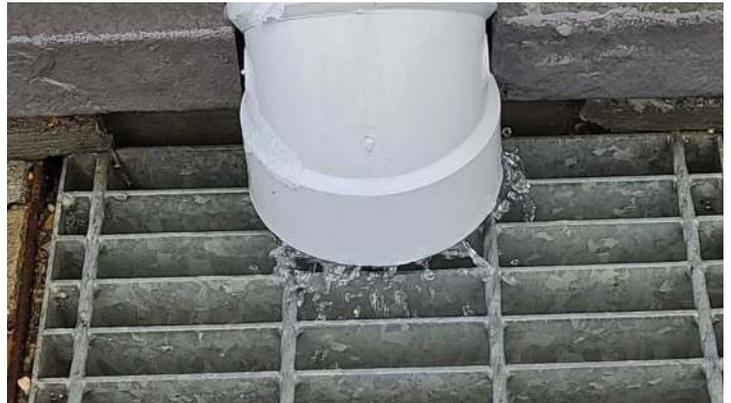
The drainage swales are clogged and leaking back towards the building, there are high levels of moisture in the concrete floor inside the building. Have a contractor evaluate and service as needed.
