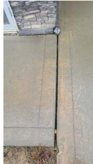
The sidewalks have typical cracks that indicate movement of the base under the sidewalk, water management needs to be addressed to control movement. If this is left it can effect the components of the building and surrounding areas.
