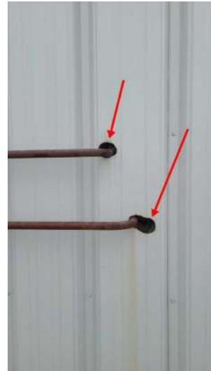
There are holes around some of the pipes in the warehouse area that need to be sealed.
