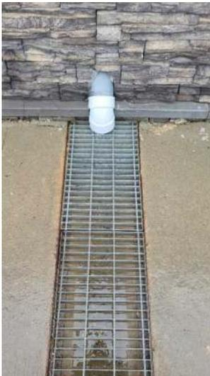
The drainage swales are clogged and leaking back towards the building, there are high levels of moisture in the concrete floor inside the building. Have a contractor evaluate and service as needed.
