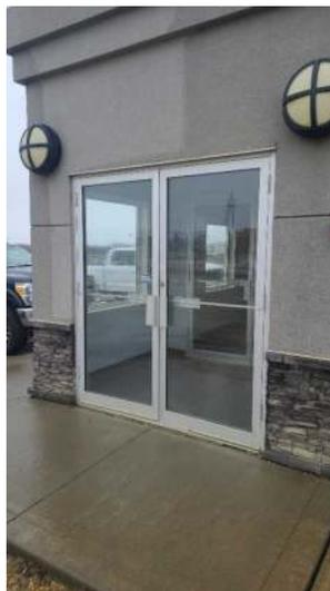
The front aluminum door does not open and will need to be serviced by a contractor.
