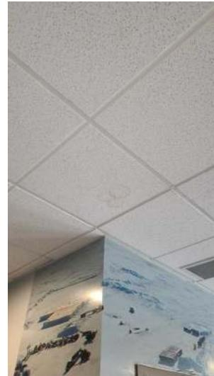
There are signs of moisture in the building that should be monitored, with the grading and drainage being poor this is a problem that may continue. A contractor should be used to evaluate the property and how to keep the moisture away from the building.
