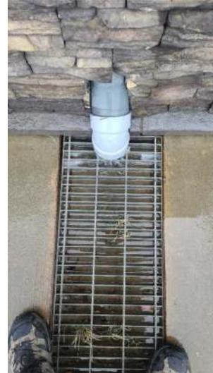
The drainage swales are clogged and leaking back towards the building, there are high levels of moisture in the concrete floor inside the building. Have a contractor evaluate and service as needed.
