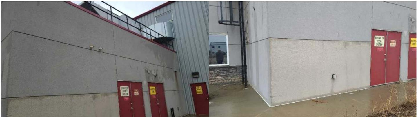
The EIFS wall covering is peeling and cracking, have a contractor evaluate and service as needed.
