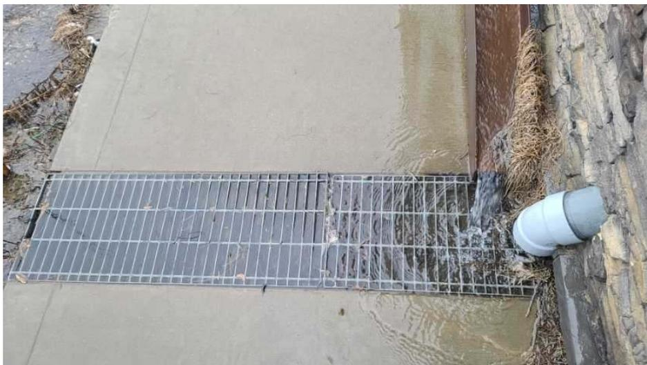
Debris blocked downspouts observed, suggest cleaning gutters and downspouts, which should be a regular part of maintenance.
