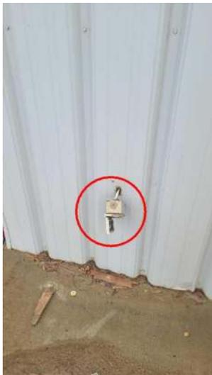
There are loose outlets on the outside of the building, have an electrician service these accordingly
